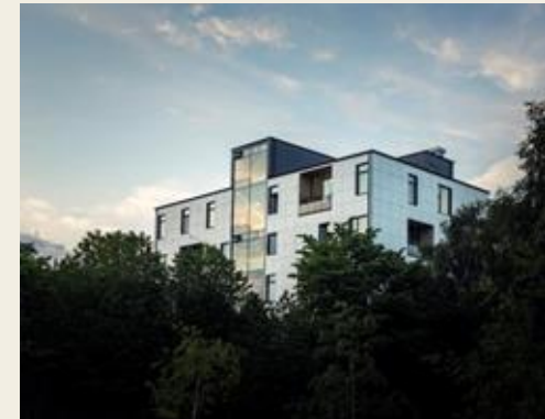
Pilot 3: Multifamily DHN connected building (Sweden)
